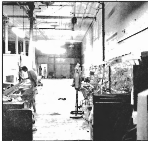
BEFORE ... renovating an old warehouse
